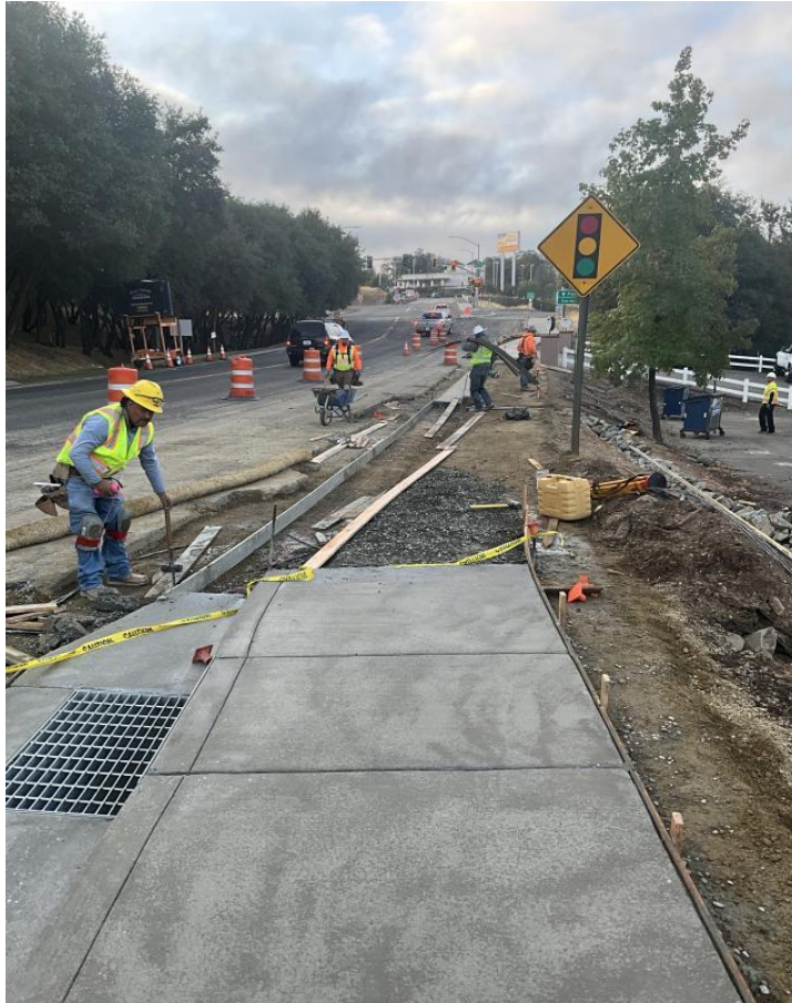
Pouring Curb, Gutter and Sidewalk
