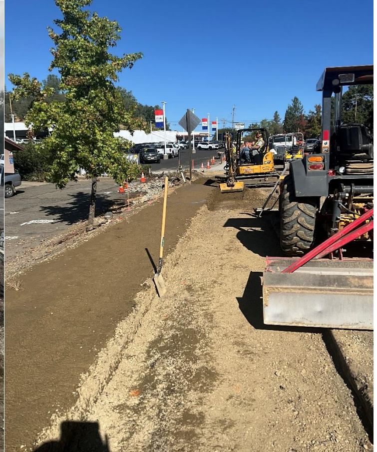
Grading for Curb, Gutter and Sidewalk
